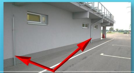
Use the lightning conductor for grounding Wire between exhaust and lightning conductor is enough.
